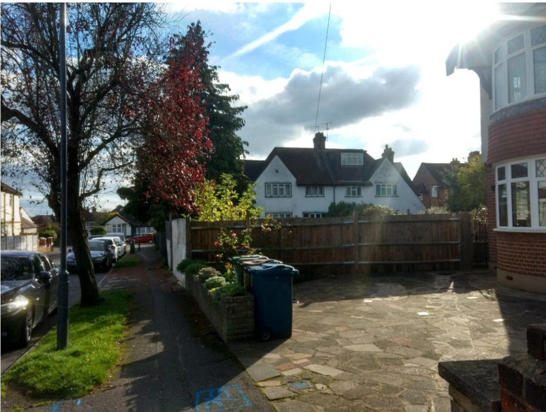
Rear elevation of subject site when viewed from Park Rise
